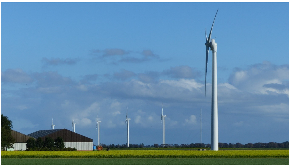
Windturbines in de Wieringermeer
